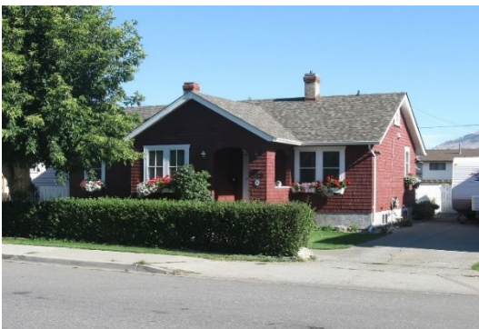
strong wooden frame structure with brick veneer
