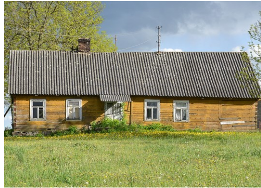
wood log (load carrying) building structure
