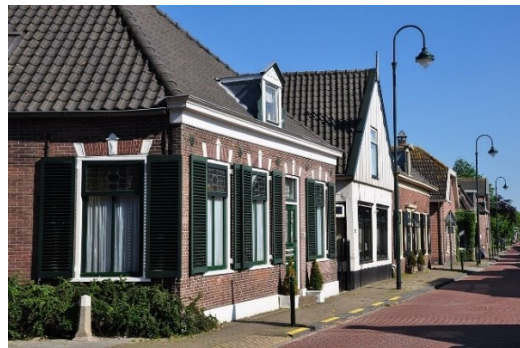
brick masonry mass wall structure
