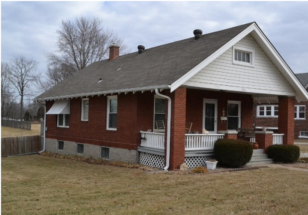
weak wooden frame structure with brick veneer
