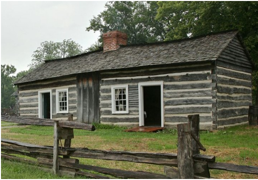
wood log (load carrying) building structure
