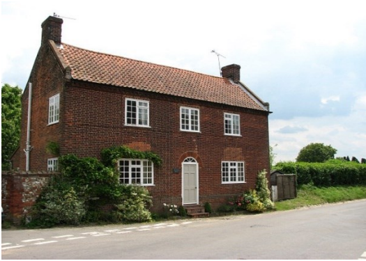
brick masonry mass wall structure
