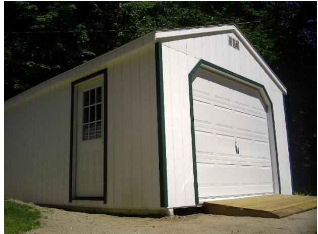
metal frame structure with wooden panels
