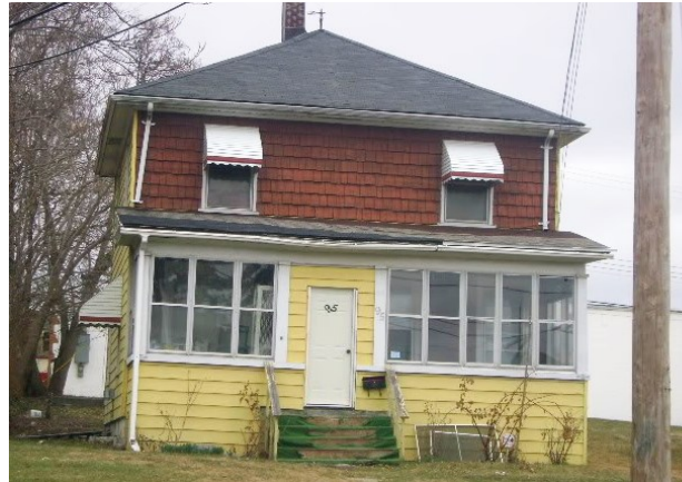
weak wooden frame structure
