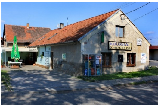
concrete block mass wall structure
