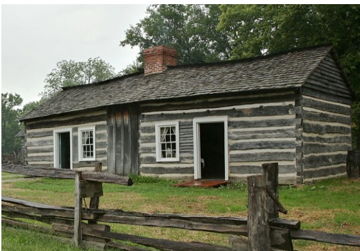
wood log (load carrying) building structure
