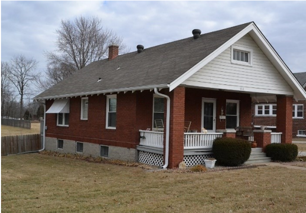
weak wooden frame structure with brick veneer
