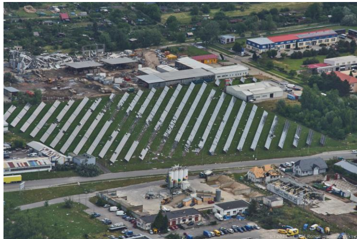
Aerial photo showing damage to the photovoltaic panels east of Lužice. Photo: Lukáš Ronge.
