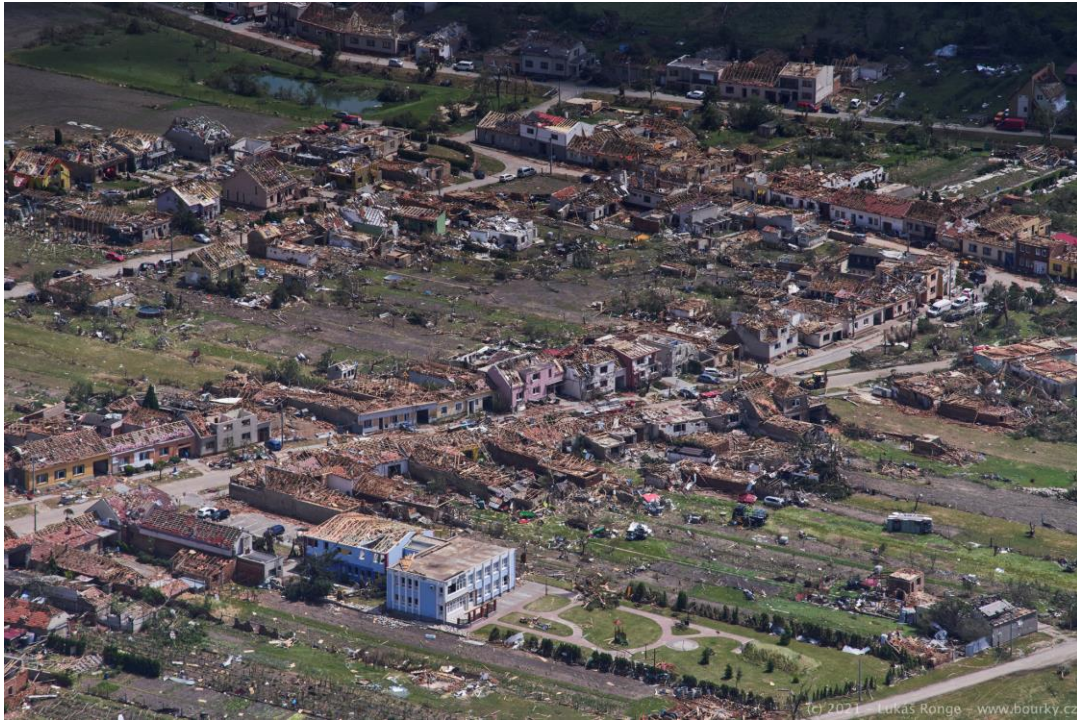
Aerial photo of significant damage in Hrušky. Photo: Lukáš Ronge
