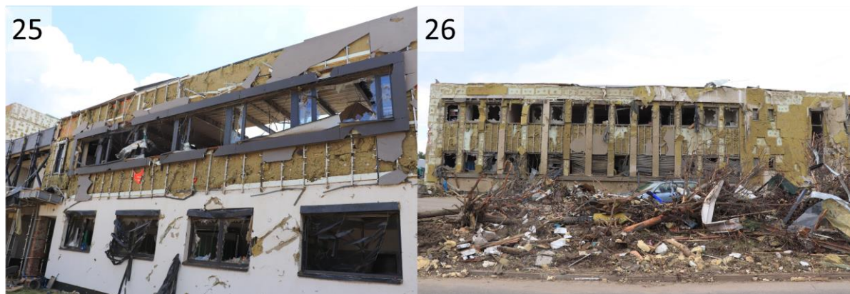
Photos showing damage in the industrial park in western Lužice. The locations of photos 25 - 26 can be found on the map of Lužice. Photos: Tomáš Půčík.
