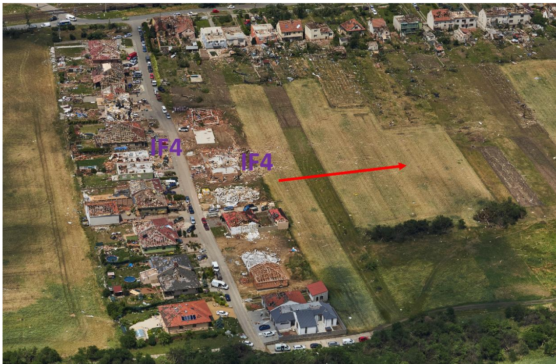
Aerial photo showing the location of IF4-rated houses in western Mikulčice and the direction of debris fall. Photo: Lukáš Ronge.
