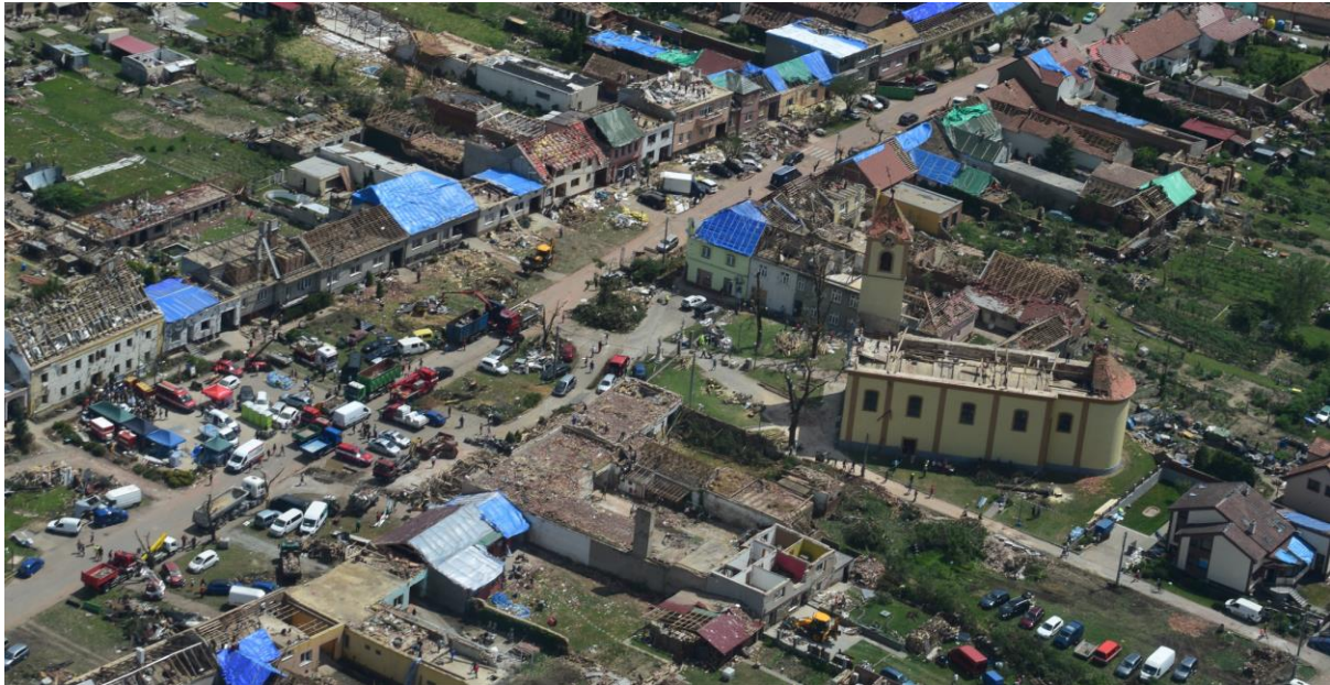
Aerial photo showing damage to the central part of Moravská Nová Ves. Photo: Miloslav Staněk.
