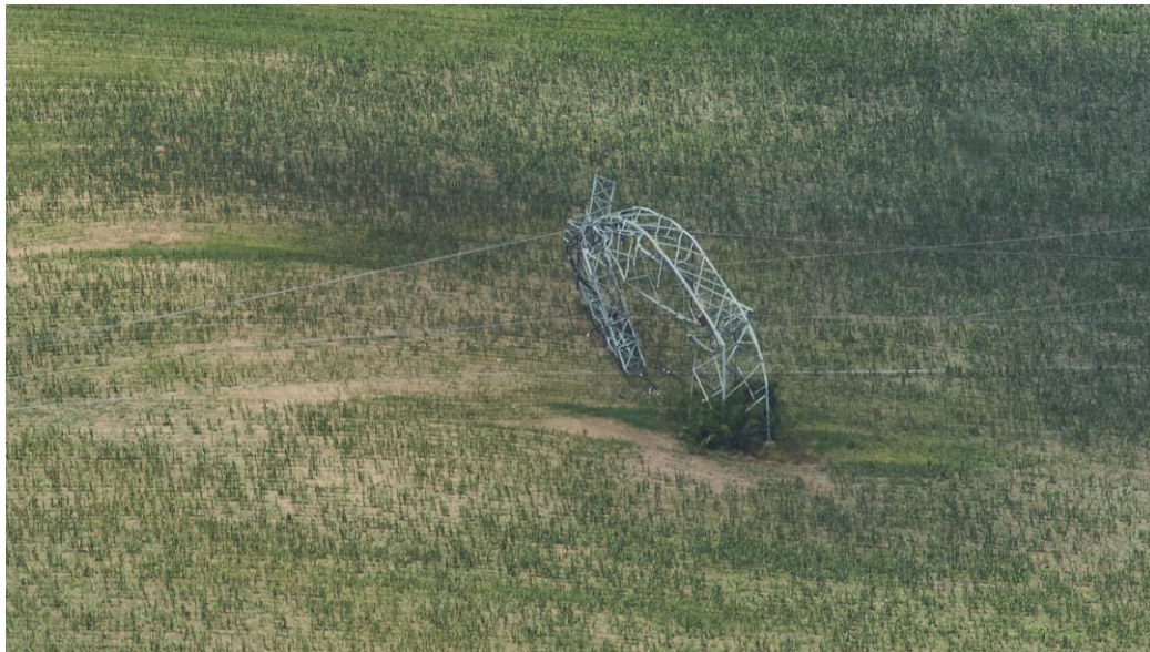
Destroyed pylon of 400 kV power lines. Photo: Lukáš Ronge
