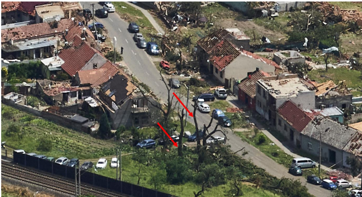
Aerial photo showing the vegetation and roof damage in western Mikulčice. Arrows point at the debranched trees with an IF3 damage rating. Photo: Lukáš Ronge.
