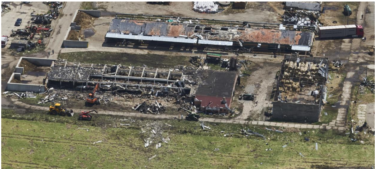
Aerial photo showing significant damage to the cattle pen with the collapse of some of the concrete walls. Photo: Lukáš Ronge
