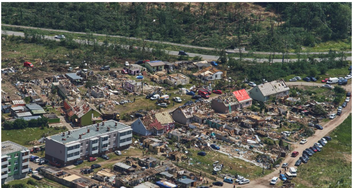
Aerial photo showing the damage in Pánov. Photo: Lukáš Ronge.
