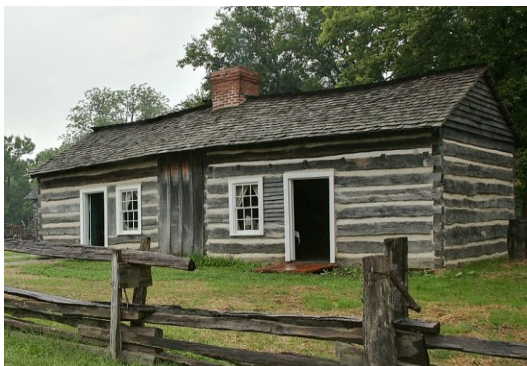
wood log (load carrying) building structure
