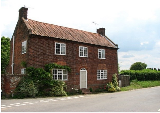
brick masonry mass wall structure
