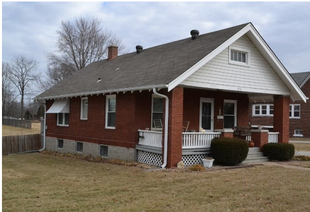
weak wooden frame structure with brick veneer
