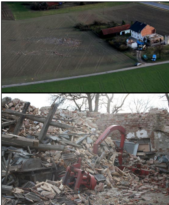
FIG. 3: Examples of the storm damage as seen from the helicopter (top) and at the surface (bottom).
