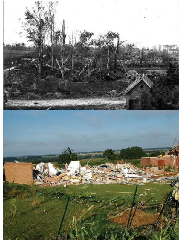
FIG. 4: Violent tornado damage (T8/F4 – 335-377 km/h); upper part: 01.06.1927 - Auen / Germany (Photo: Heinz Brinkmann), lower part: 03.08.2008 - Hautmont / France (Photo: Bjoern Stumpf).
