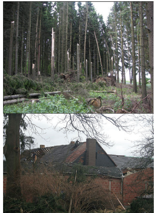
FIG. 2: Weak tornado damage (T3/F1 - 151-183 km/h); upper part: 29.05.2007 - Borler / German (Photo: Erik Dirksen), lower part: 01.03.2008 - Uttershausen / Hessen (Foto: Eyk Neidert)
